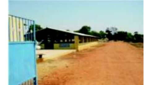
Waste Management Centre
